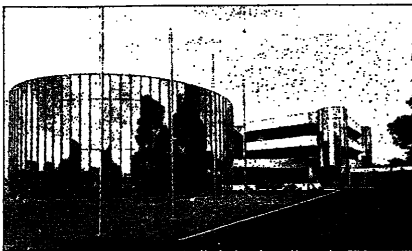
A computer controlled visual, audio and climatic environment. Only with electricity.
